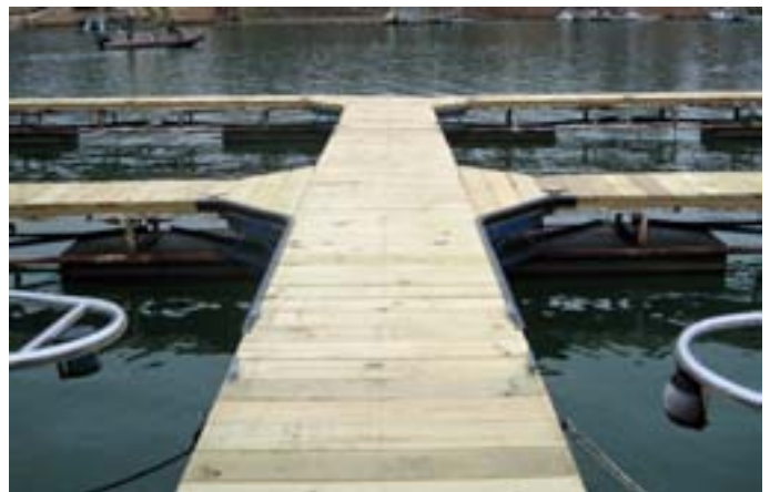
End Section, Dock 2, New Decking
